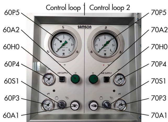
Fig. 7: Type 7311-01/-02/-03 Air Control System with connections
